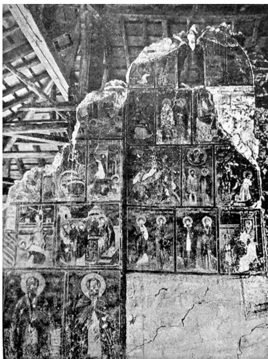
Fig. 18. The West façade of the gallery of Sts. Peter and Paul's Church in Veliko Tarnovo after the earthquake in 1913 (the personal collection of I. Panayotov).
